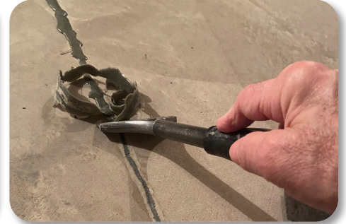
Shave in less than 60 minutes and install immediately over joint. Less time to install flooring vs. patch
