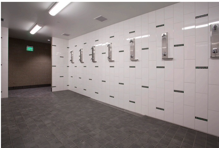
TEC® InColor™ can be used in submerged areas, such as swimming pools, showers and fountains. Allow seven days before full water submersion.
