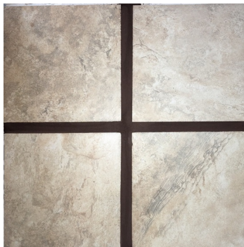
Figure 24 TEC® Power Grout® (Espresso) grout sample before efflorescence emittance test
