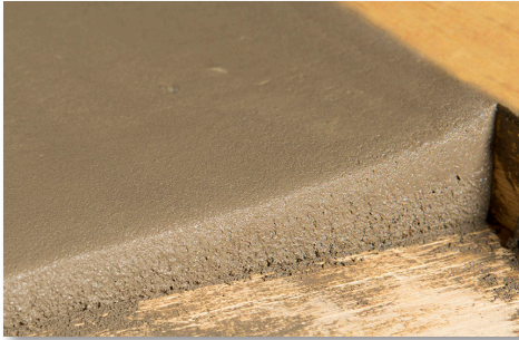
Ramping Apply up to 1½" thick in a single application
