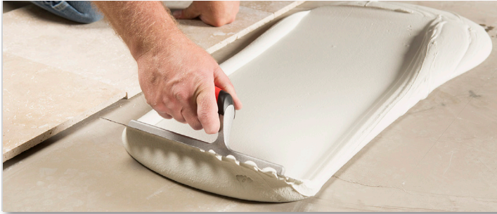
Can be used for bedding thicknesses of \frac{3}{32} " - \frac{3}{4} " (2.4 mm - 19 mm)
