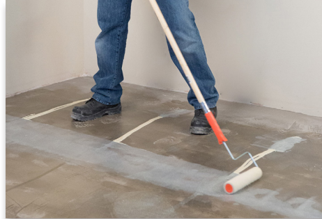
Roller-applied adhesive allows installer to roll the adhesive onto the substrate efficiently
