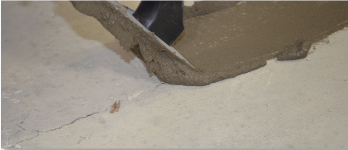
Can be applied to concrete with a relative humidity (RH) up to 90%
