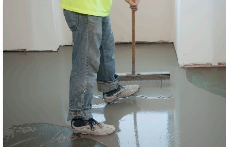
Single applications from 1/8" to 2" (3-50 mm) neat
